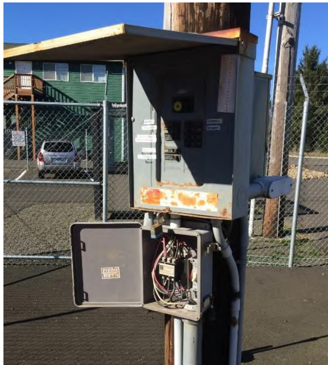
Figure 3: Existing Electrical Panel to be Replaced by Electrical Building
